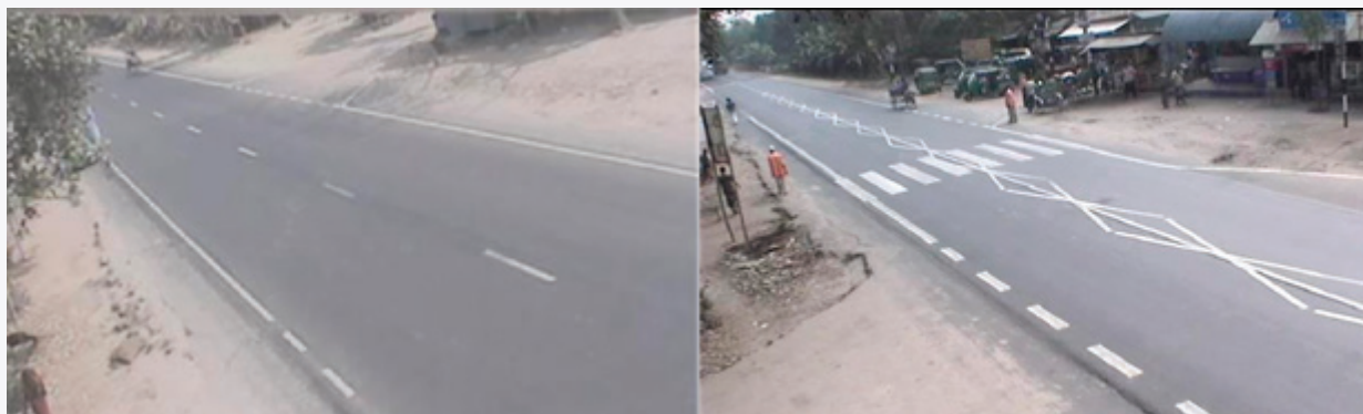
Before and after the infrastructural interventions. Speed hump is located 60 m from pedestrian crossing. © van der Horst
